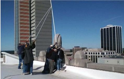
The feedline and a grounding system were then added. A check of the VSWR indicated essentially no return power, characteristic of a satisfactory VSWR and thus antenna install.
